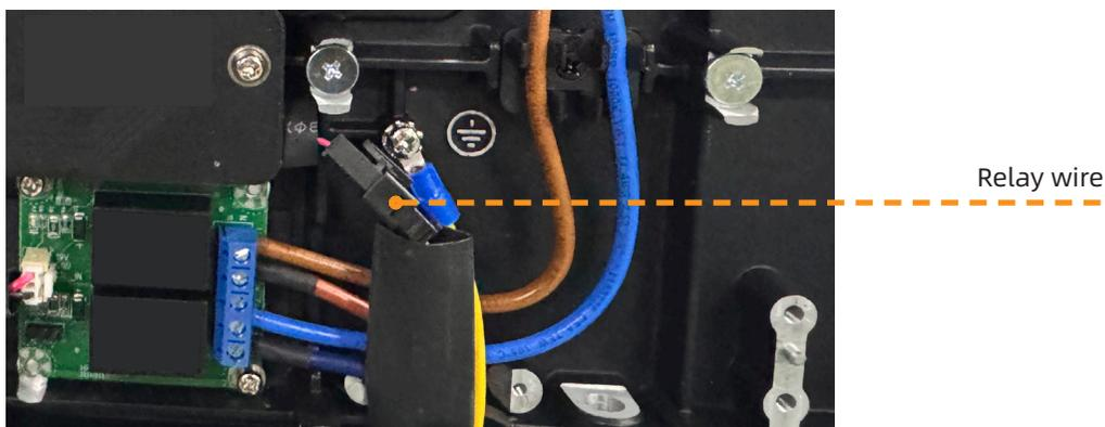
**Step 3.** Connect the power lines, numbered Line 1-6, to the F1-A1 cabinet in sequence:
