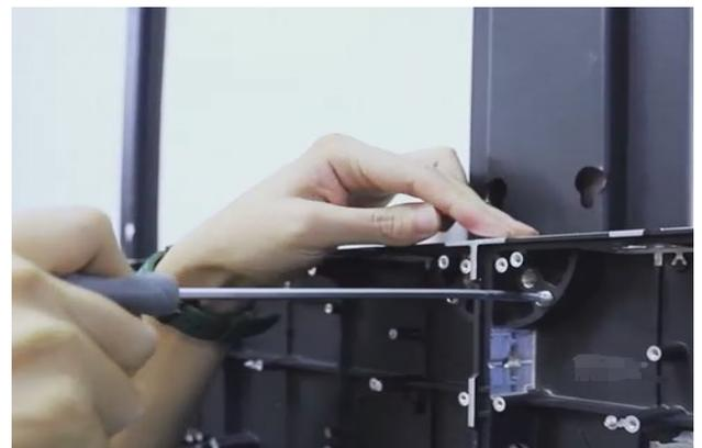
4. Secure the cabinet in the larger hole with set screws, then use a hex socket wrench to tighten the screws and mount it onto the bracket
