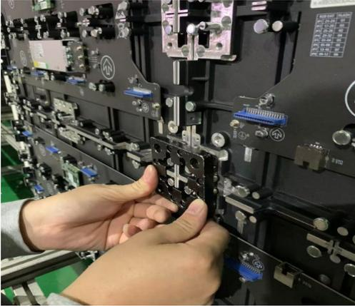
5. Install the front connecting piece between the cabinets.
