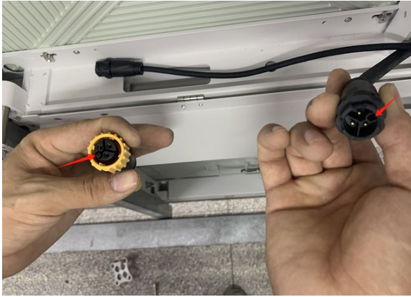
8.Align the holes and connect the power cables.
